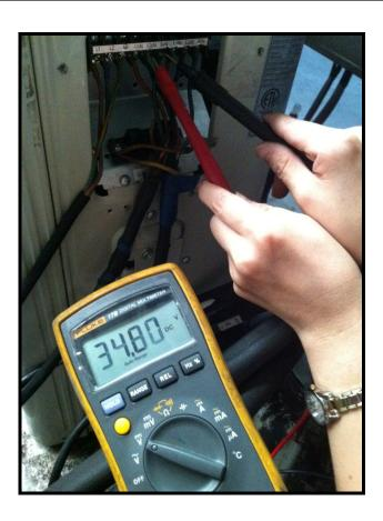
Pic 1: Use a multimeter to test the DC voltage between 2(old: L2) port and S port of outdoor unit. The red pin of multimeter connects with 2 (old: L2) port while the black pin is for S port.
